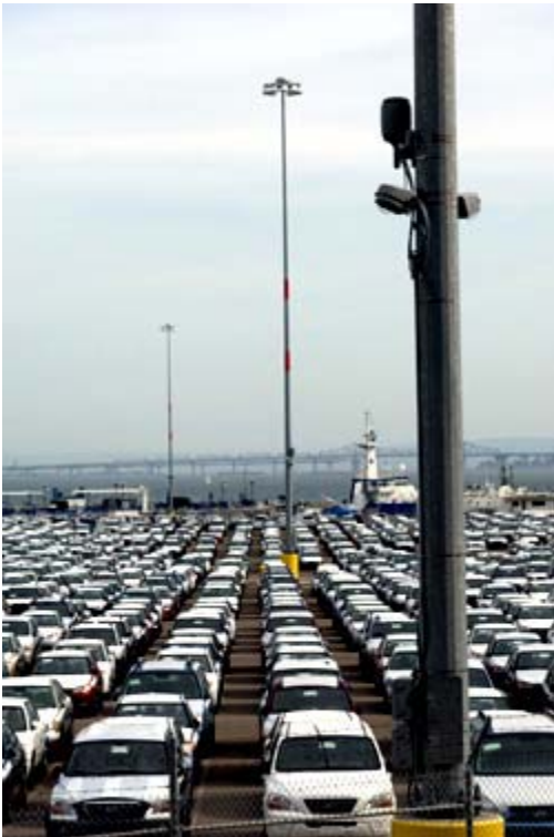
CAPTION: Two pan-tilt-zoom cameras and a BelAir 200 unit overlook a car unloading area at the Port of Richmond. Each camera is supported by a minimum 2 MB of bandwidth at all times.
