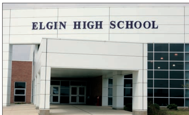
Elgin High School, located just east of Austin, Texas, recently teamed with ADT Security Services to design and install a 22-camera security system with a digital video recording system.
